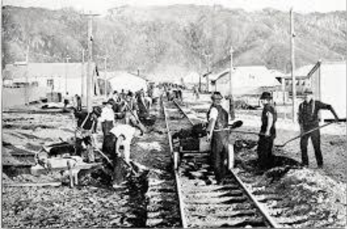
WORKERS AT THE RAILROAD TRACKS IN THE MOUNTAIN REGION OF MONTANA. THE TRACKS ARE BEING BUILT BY THE GREAT NORTHERN RAILROAD COMPANY.
